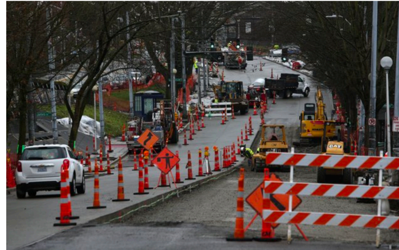
The rebuilding of 23rd Avenue in Seattle's Central District is among the projects that benefited from the Move Seattle transportation levy. (Ken Lambert / The Seattle Times)
